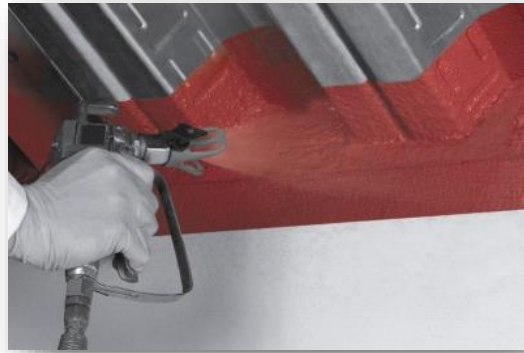
Metal Deck Joints
