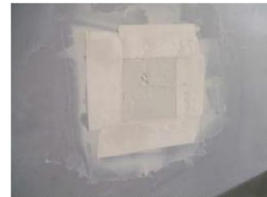
Figure 5: Tape and Finish Patched Area
