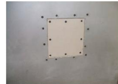
Figure 4: Apply Gypsum Panel Patch
